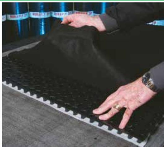
Drainage mat laid on membrane
