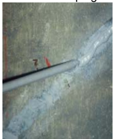
Capping cracks
