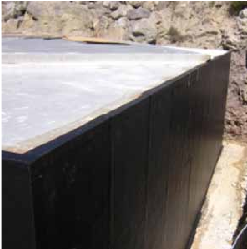
Typical waterproofing using Shelterseal 3000X
